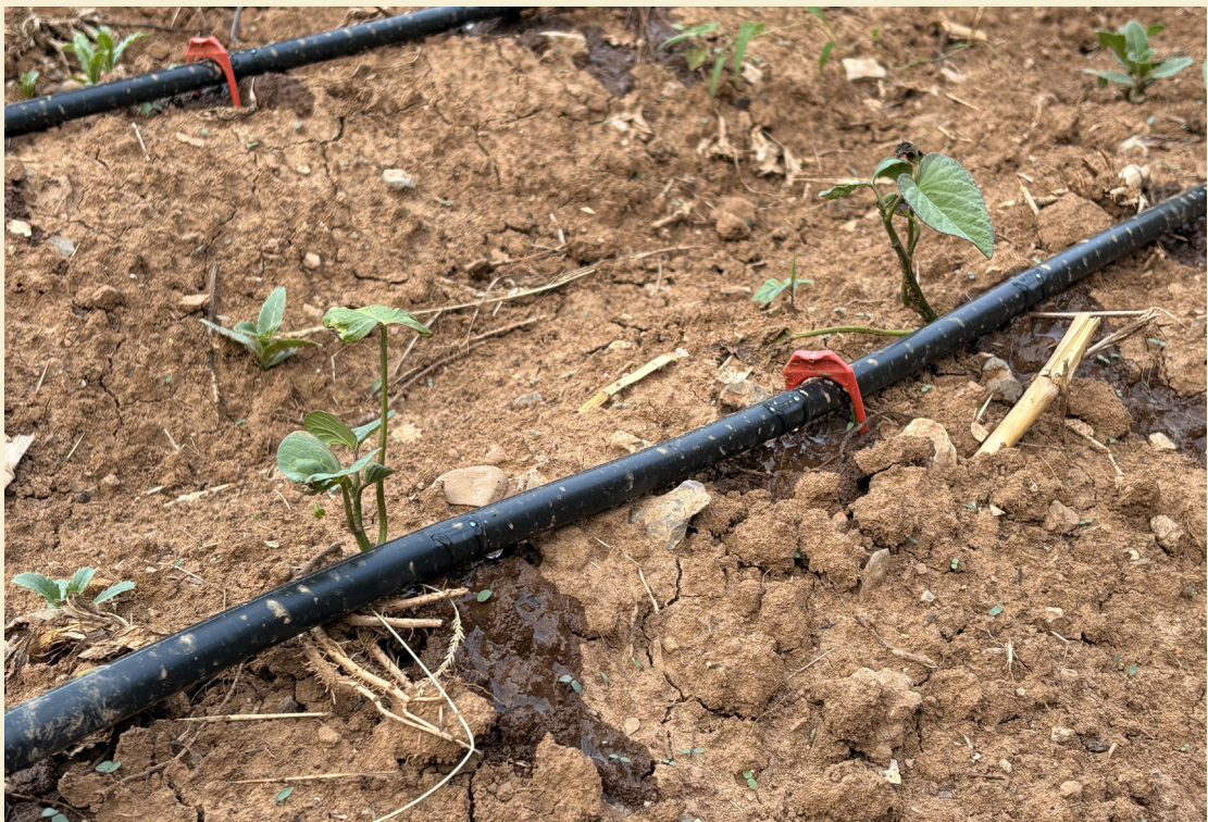
The water cellar plus drip irrigation system installed in Wangjinzhuang is both water-saving and precise in irrigation, which enhances the utilization efficiency of water cellars.
